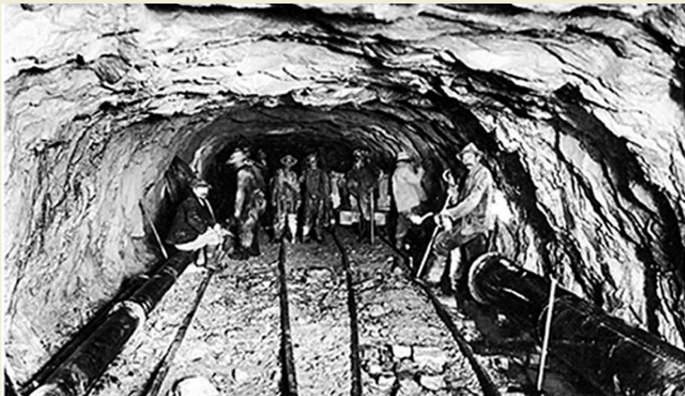
14.6 km of the Lötschberg tunnel in Switzerland (13,735 m) was largely dug by hand
